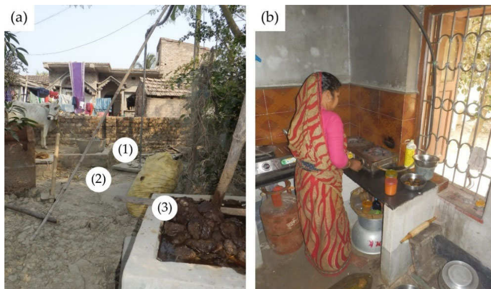
Figure 7. Household biodigester (a) Deenbandhu Model: (1) inlet filled with manure and water; (2) underground fixed-dome fermenter, and (3) outlet chamber in the rural village of Ghoragachha, West Bengal India. (b). Women cooking on a biogas stove, directly connected with the biodigester.
